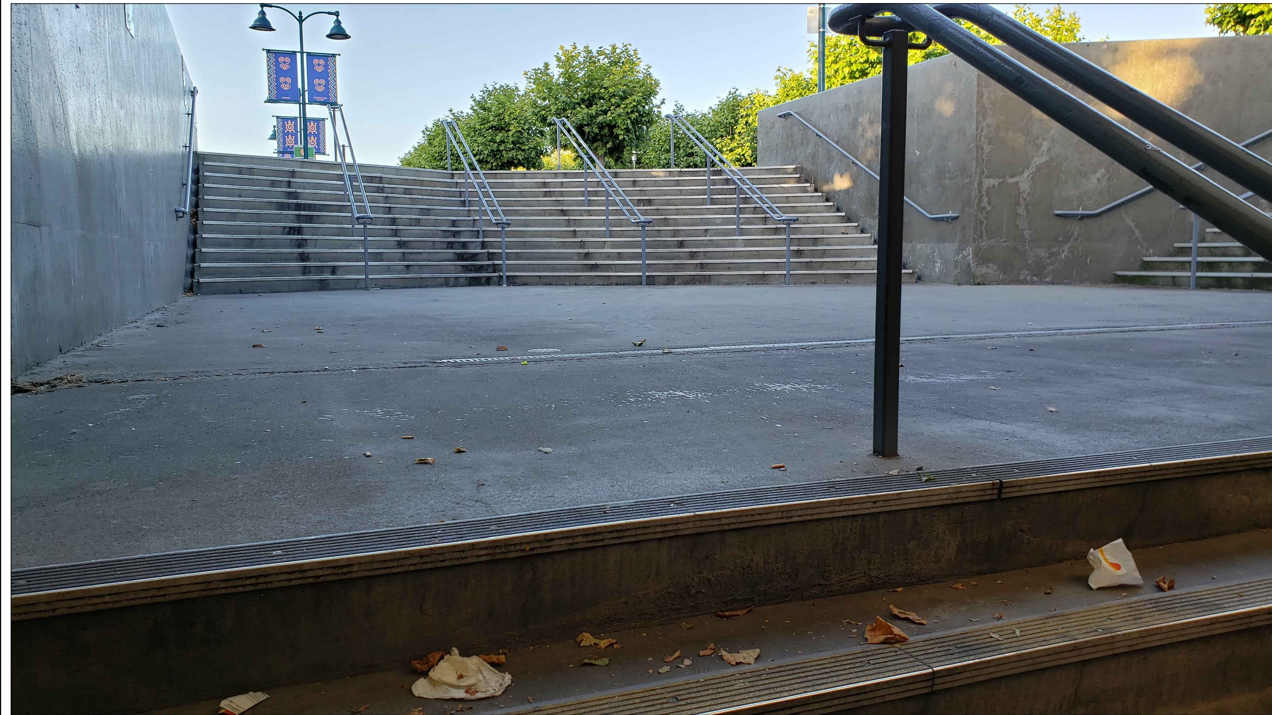
1 STAIR E2 & E4 – VIEW AT STREET LEVEL A402 SCALE:NTS
