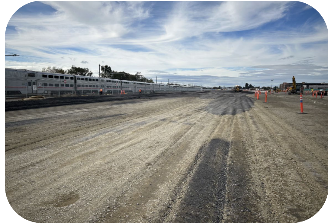
Grading complete for top of launch structure.
