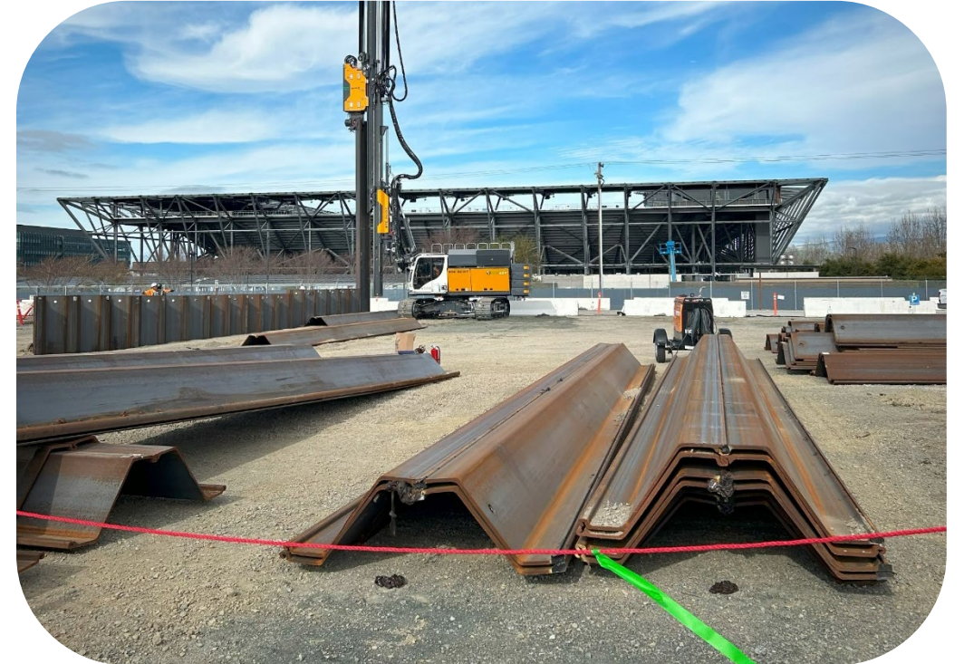
Preparing and installing sheet piling for detention pond.
