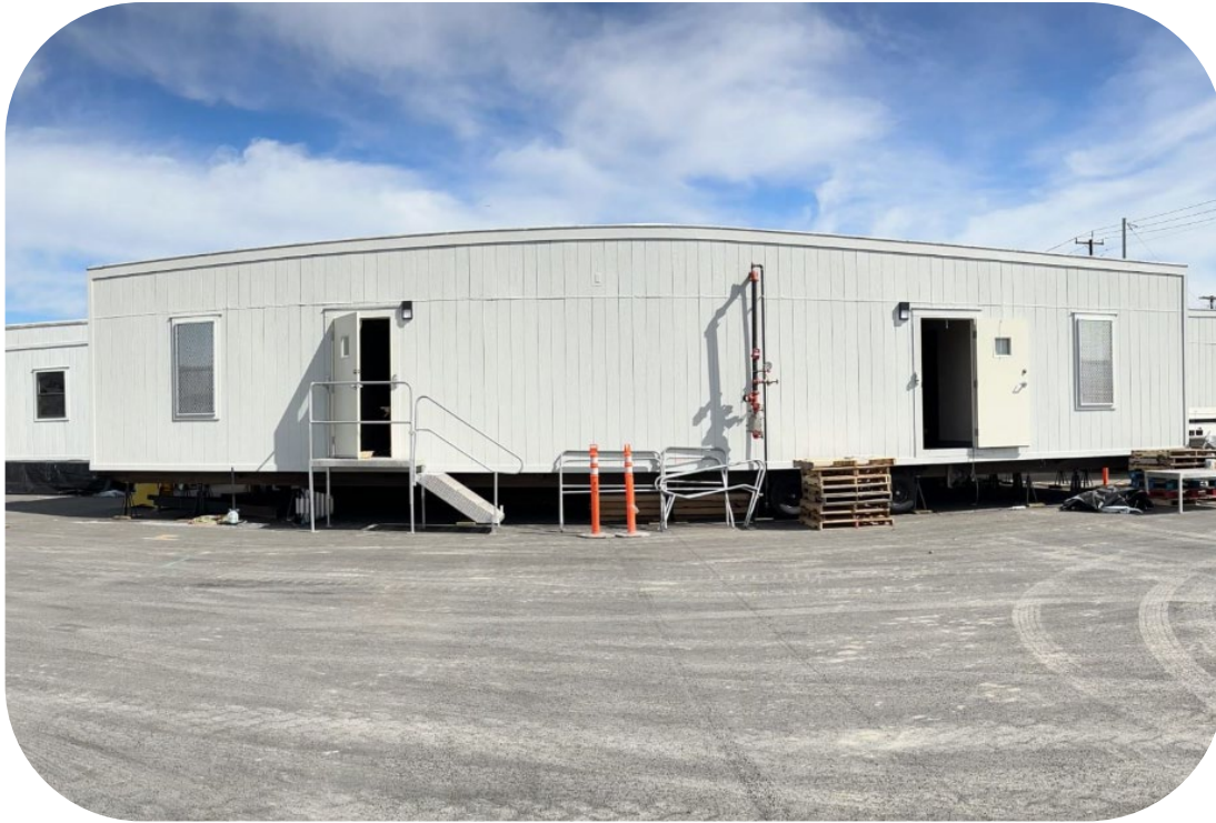
Set up and connection of office trailers on site.
