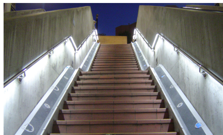
5 Expand Bicycle Access Install bicycle channels on 19th St. stairwell and increase bicycle parking in station
