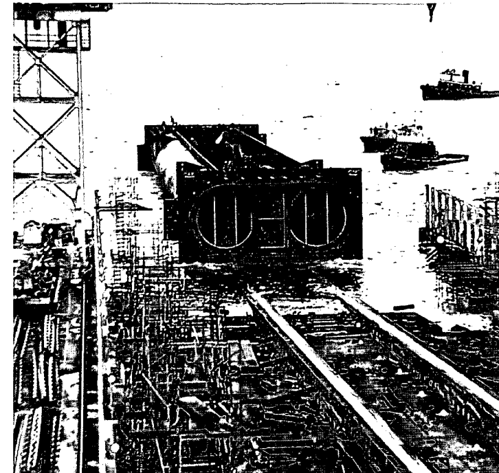
In February 1967, the first of the 57 sections used in BART's Transbay Tube was launched like a ship. The sections were towed to a nearby dock, where 4,200 cubic yards of concrete were poured in to the interior to form the 2.3 foot interior walls and track bed.
