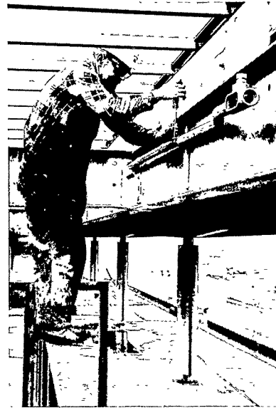
Electrician installs conduit in Richmond Station.
