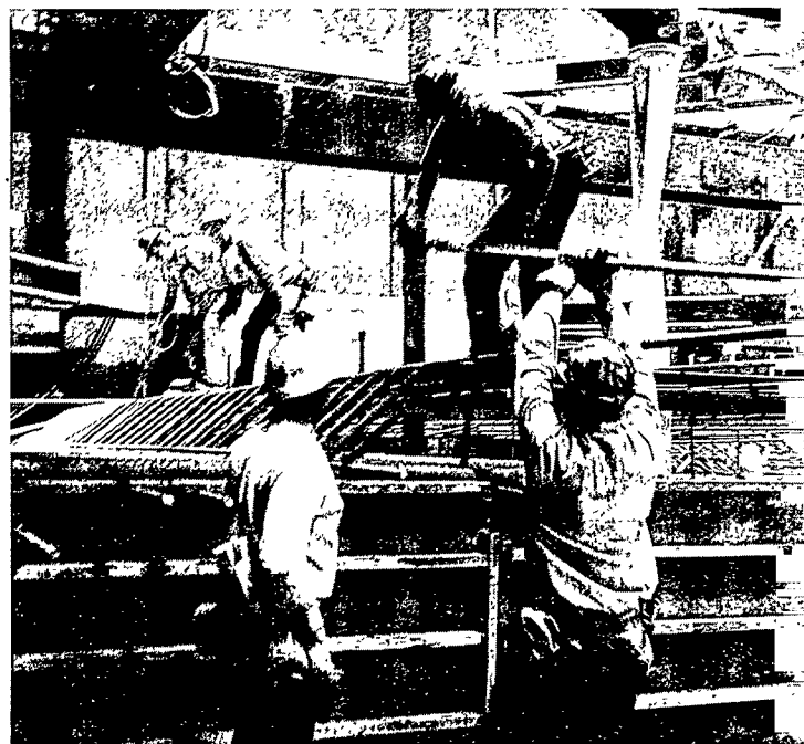
Steel men wrestle heavy re-bars into place for underground station.
