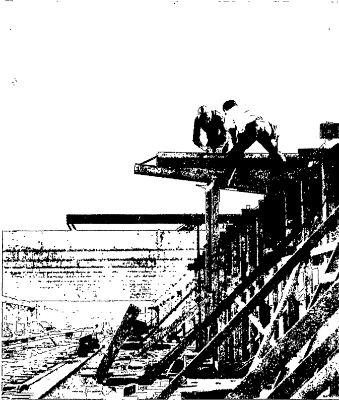
Workmen on aerial station.
