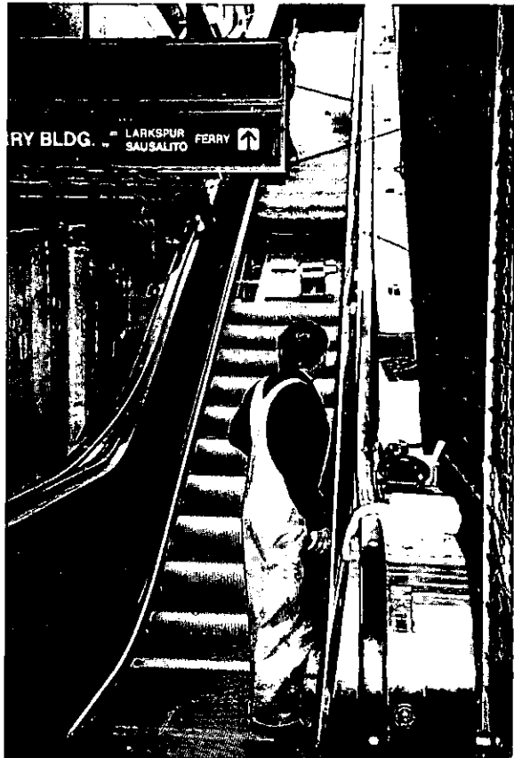
Installing Balustrade panes at Embarcadero Station.
