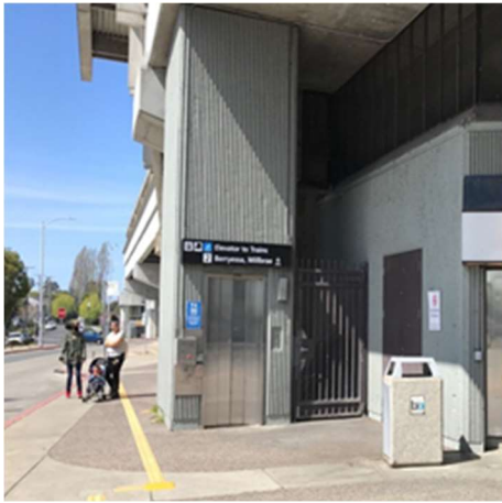
Figure 2: Exposed Elevator 1 on Concourse Level
