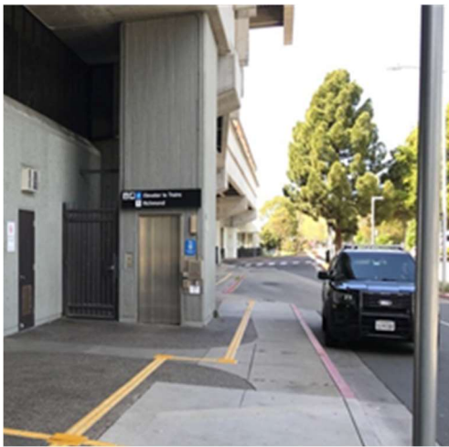
Figure 4: Exposed Elevator 2 on Concourse Level
