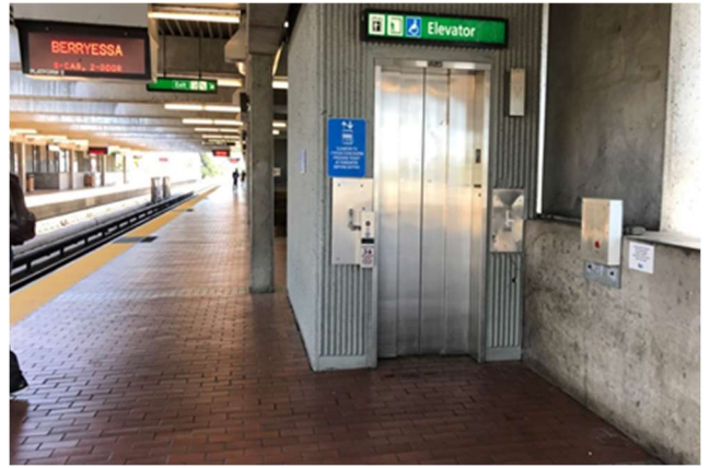
Figure 3: Exposed Elevator 1 on Platform Level
