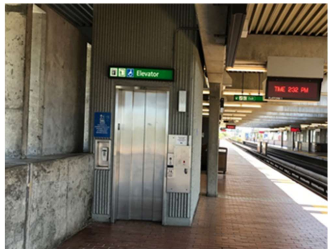
Figure 5: Exposed Elevator 2 on Platform Level
