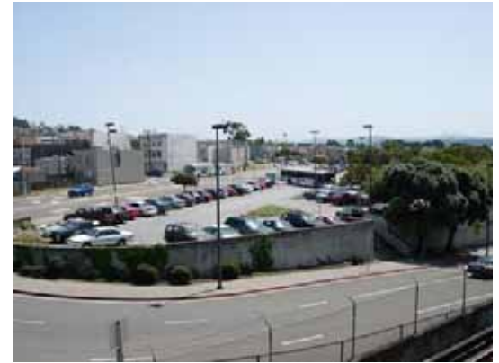
DeLong Lot: site of Transit Village and New Intermodal
