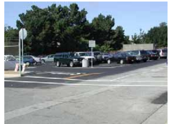
Parking Lot North of Garage
