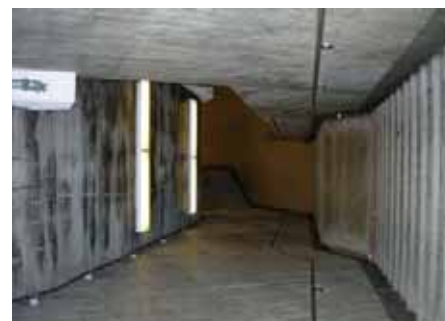
Tunnel under John Daly Blvd
