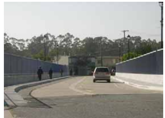
St. Charles Bridge Improvements
