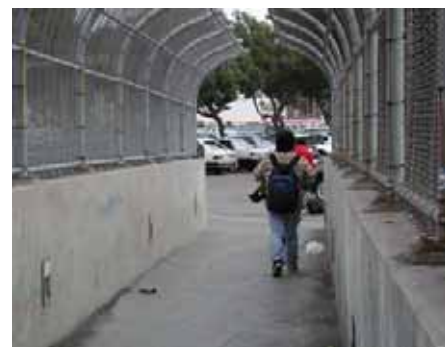
Overcrossing to Parking Lot
