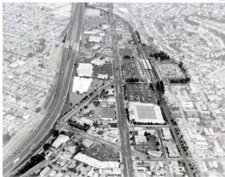
Figure 4: El Cerrito del Norte Station Area Infrastructure
