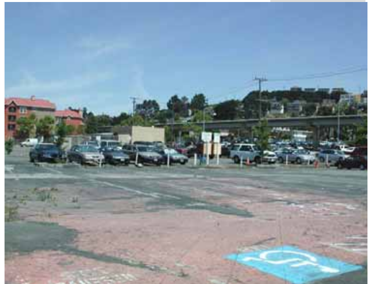
El Cerrito del Norte Station Surface Parking
