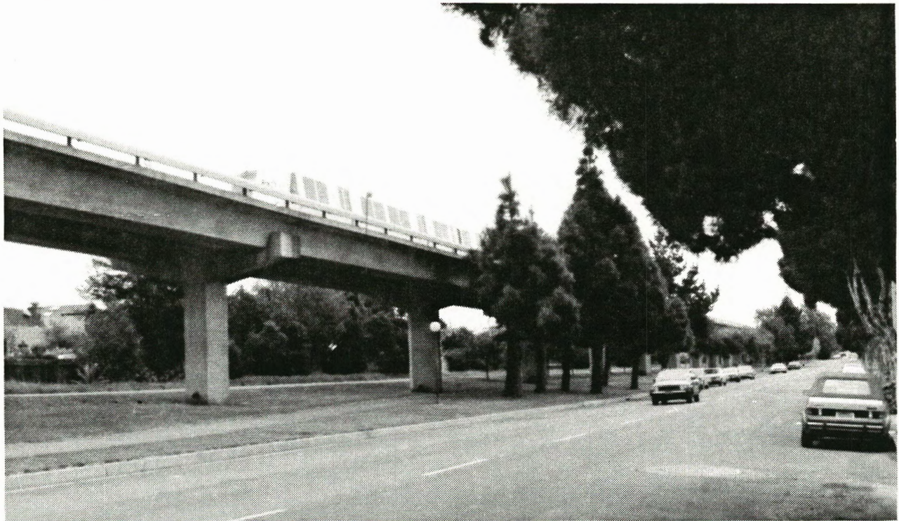
BART Aerial Structure Without Noise Barrier Wall - Richmond Line South of Marin Avenue in Albany
