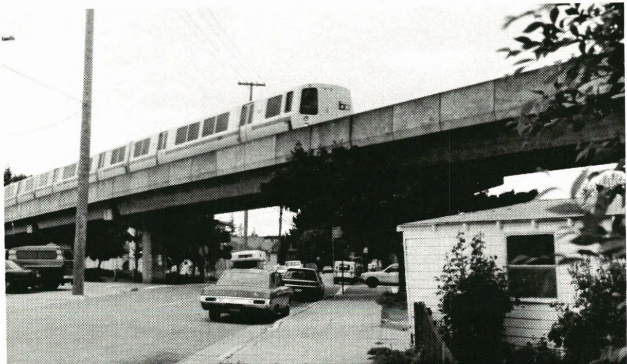
BART Aerial Structure With Noise Barrier - Richmond Line North of Gilman Street in Berkeley
