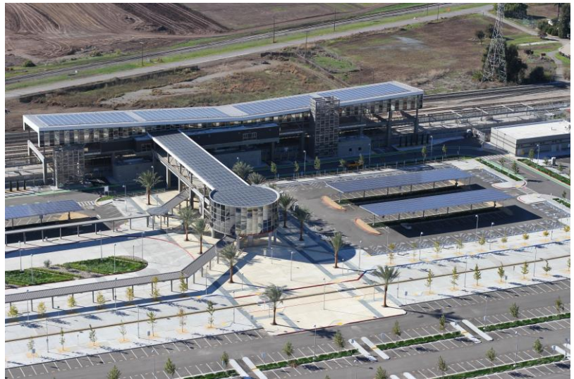
Aerial photo of new BART Warm Springs/South Fremont Station.
