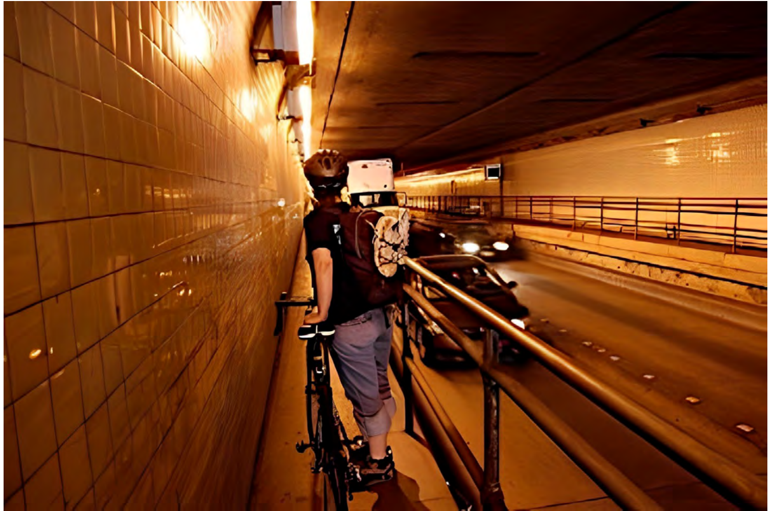
A 2009 Photo of the Underground Posey Tube Path
