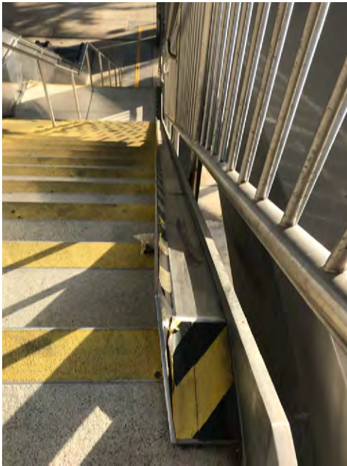
Photo is of bike channel at Warm Springs Station. Actual bike channel for Irvington will follow latest design.
