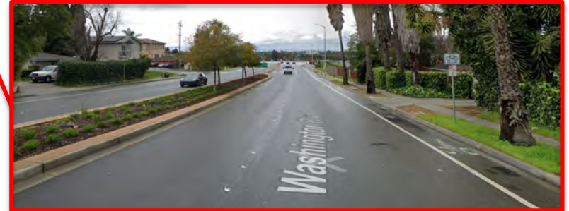
Washington Blvd Class II Buffered Bike Lanes (Future Upgrade to Class IV Separated Bikeway)
