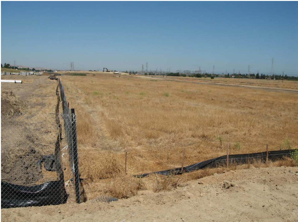
Photo 1: View of the proposed staging area looking west from the Maintenance Facility. SR 4 construction is visible left of the fence. Equipment visible in the far background is the parking lot construction.
